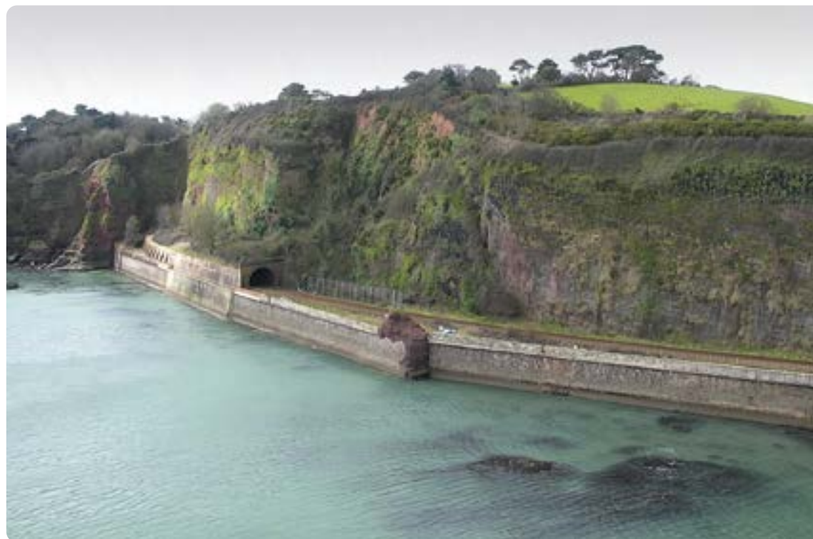
Source: Network Rail
