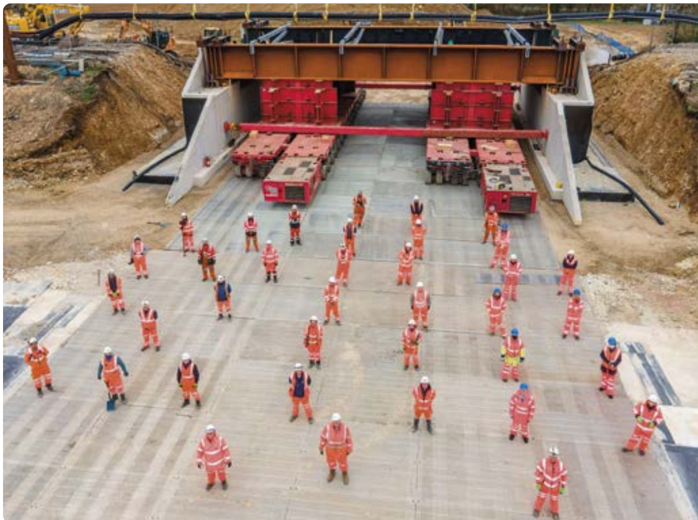
Source: Network Rail
