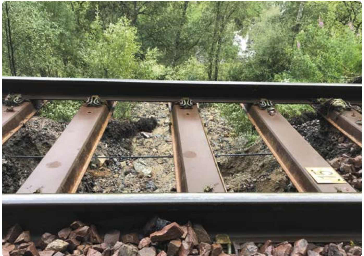
Source: Network Rail
