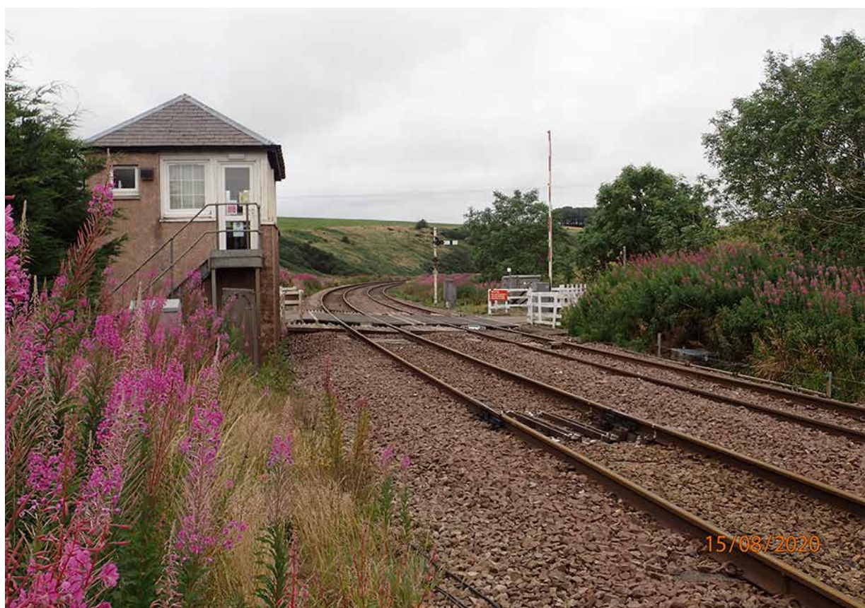
Figure 57: Carmont signal box looking north
