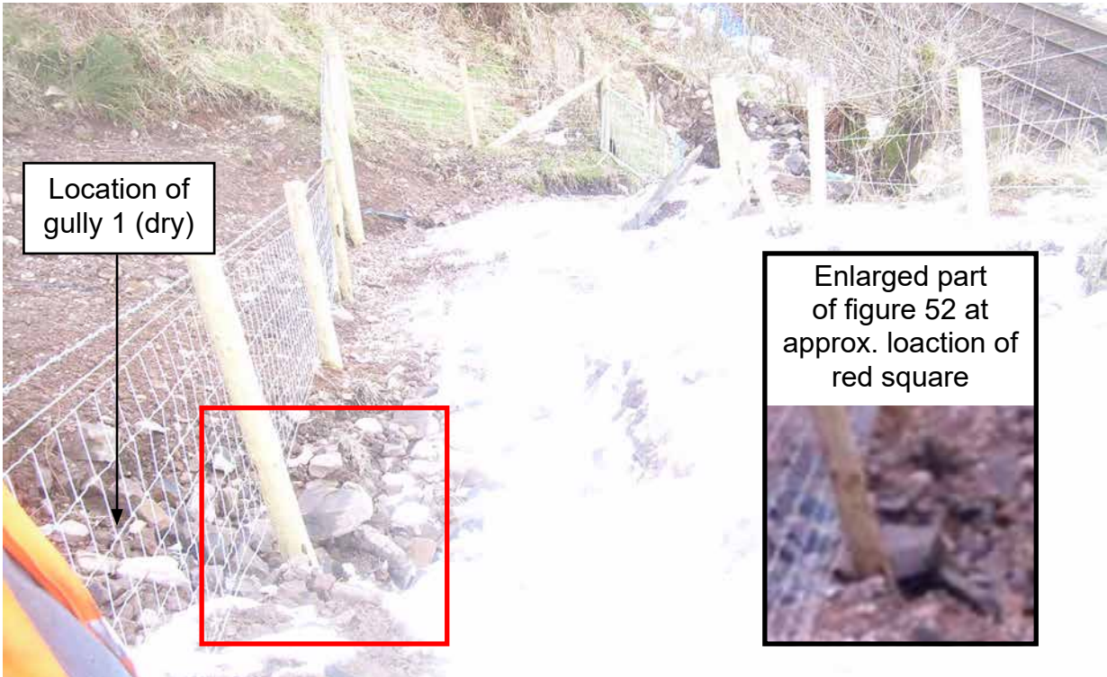
Figure 53: Surface of drain in light snow looking towards CP18 and railway in March 2013 during an inspection of the completed works (Network Rail). The original image is over-exposed
