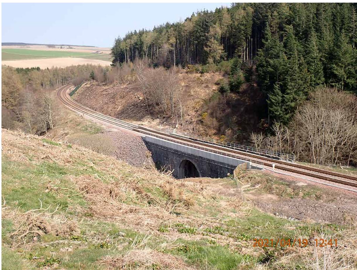
Figure F.9: Bridge 325 in April 2021 following the replacement of the down-side parapet and track
