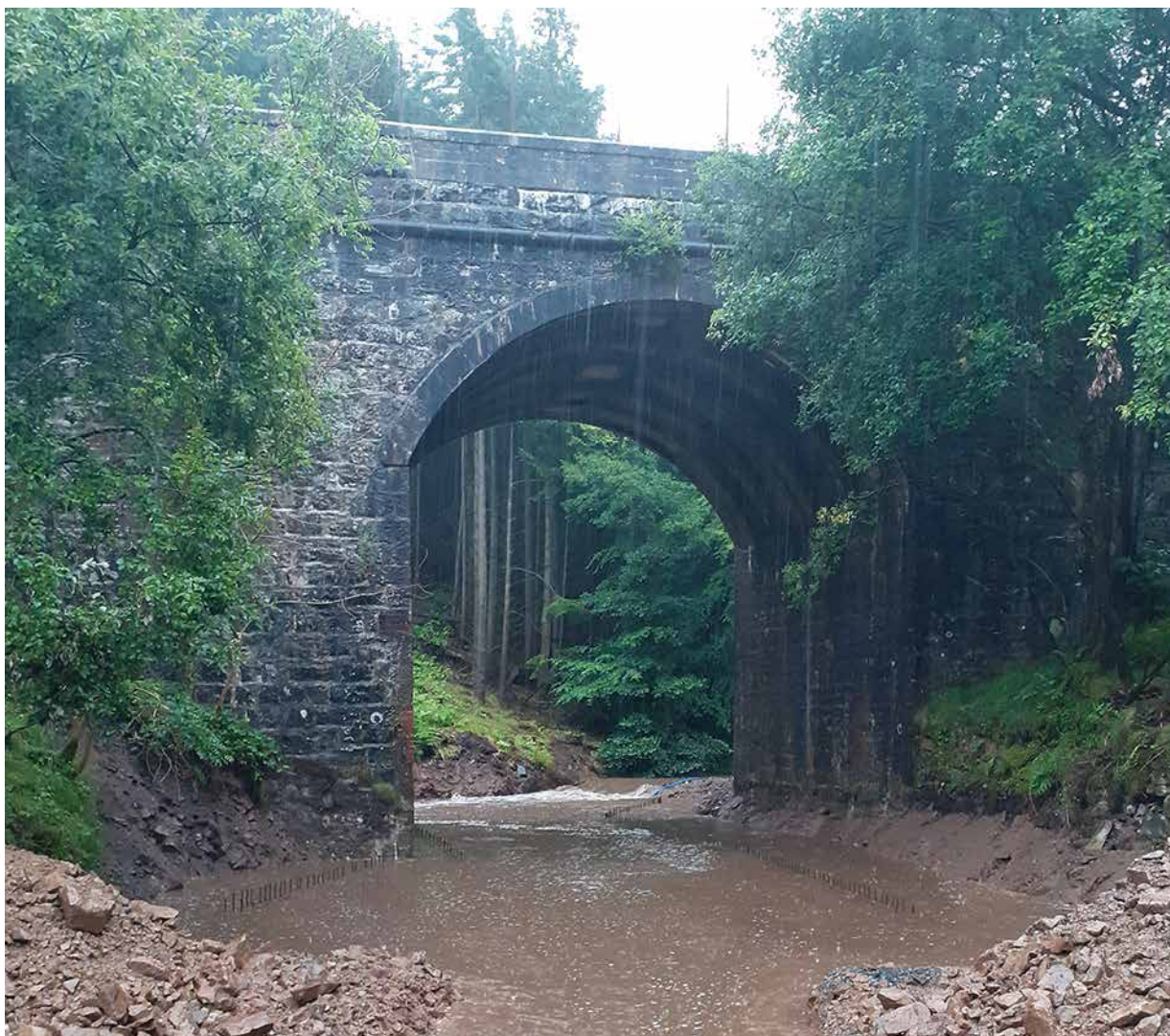
Figure F.4: Down-side elevation of bridge 325 at 08:19 hrs on 12 August 2020, shortly before the accident (Story Contracting)
