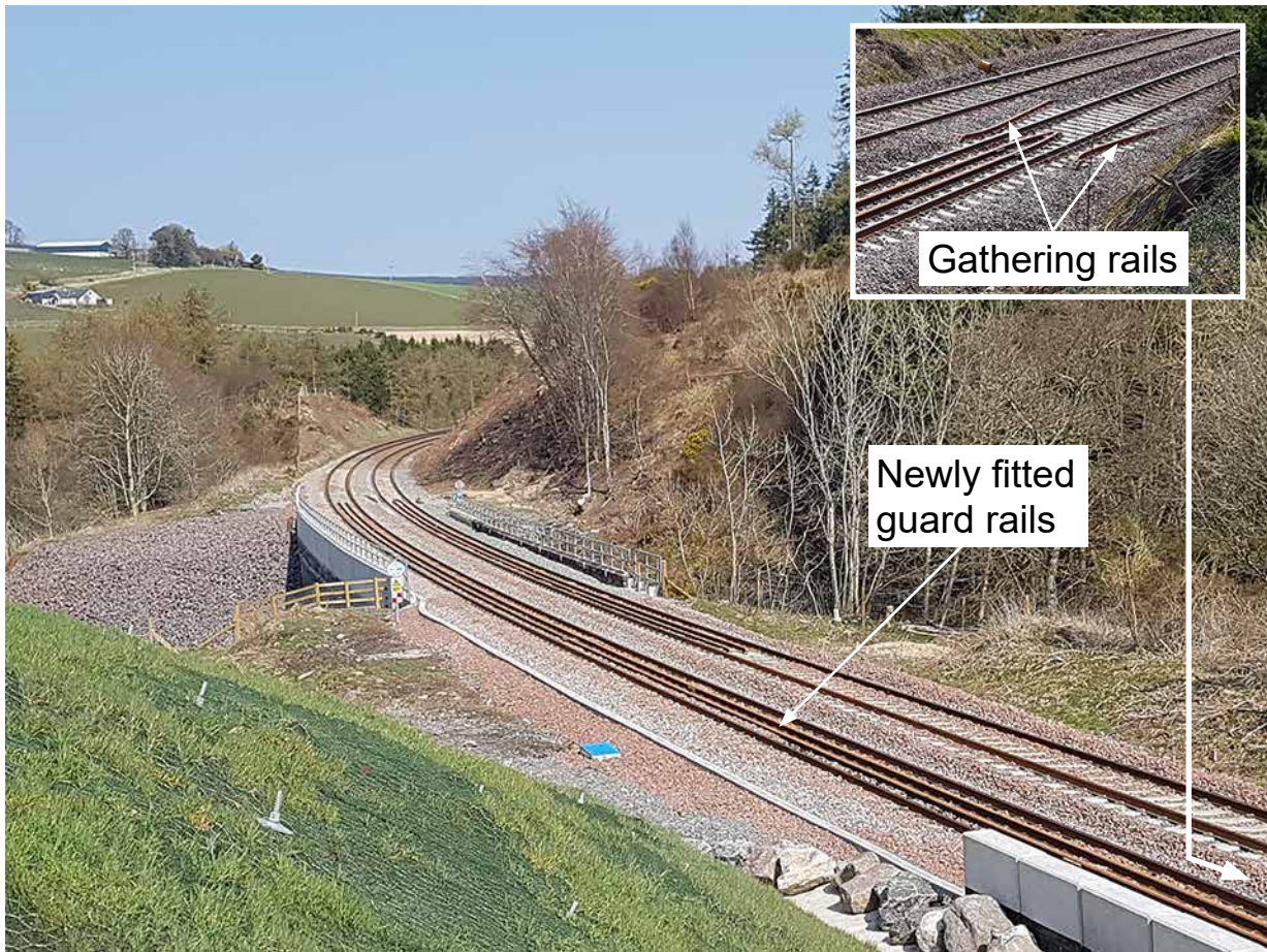
Figure 86: Guard rails fitted post-accident at bridge 325. The gathering rails are positioned at the start of the guard rails to the right of the main picture
