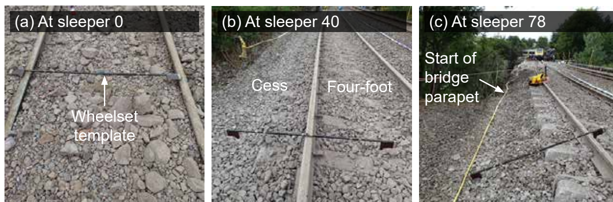
Figure 24: Position of leading wheelset (shown by wheelset template) from washout to bridge 325
