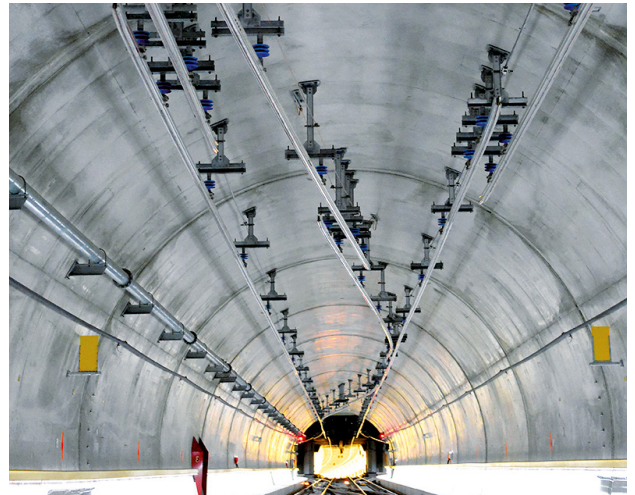
TracFeed® OSS Overhead conductor rail
