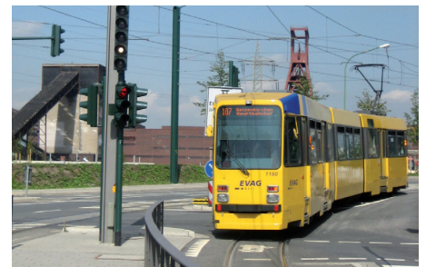
Catenary systems – with architecturally adapted design
