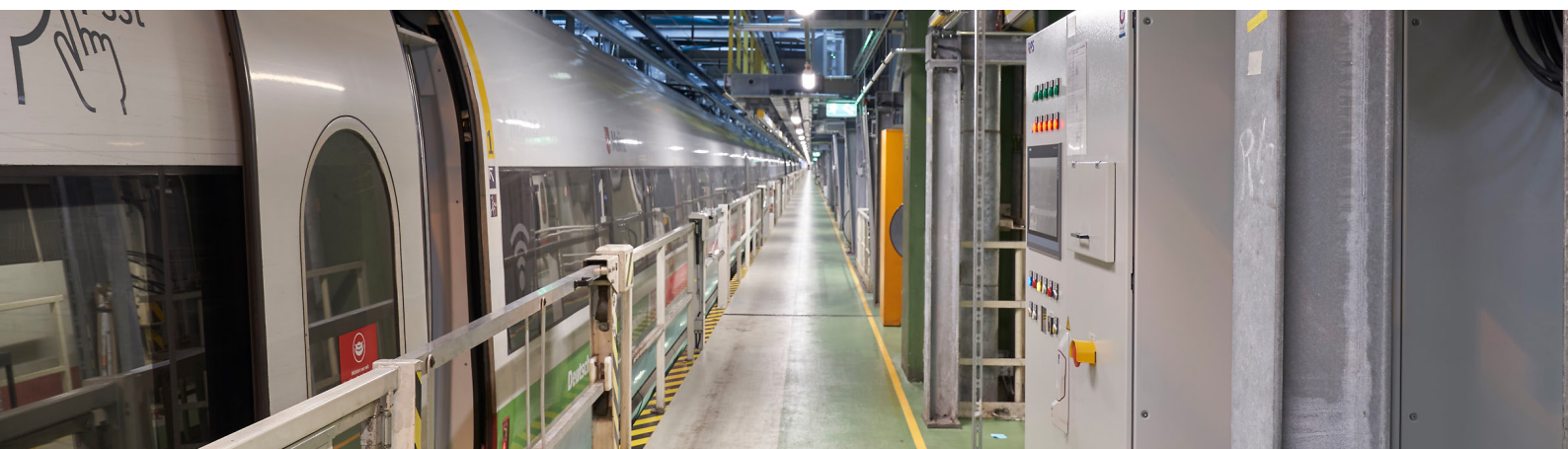
TracFeed® AEA – assures the switch off and earthing of the catenary before work is begun
