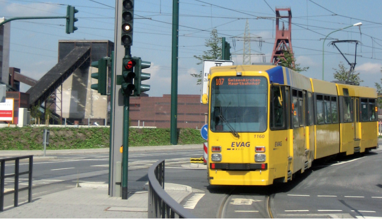
Contact line systems - designed as overhead line
