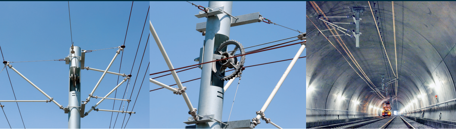
Assembly Stuttgart Zuffenhausen - TracFeed® ALU 1000
