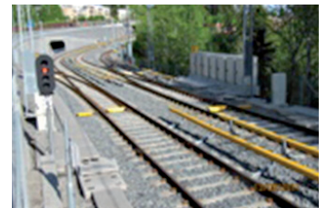
Ramps at Turnouts
